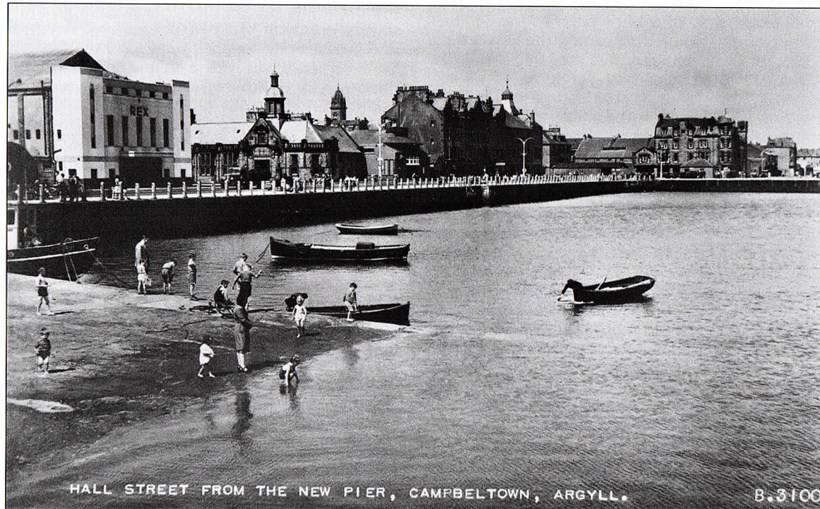
The Rex stood some 50 metres to the south of the Picture House on Hall Street. The listed library and museum came between. (Stenlake Collection.)
