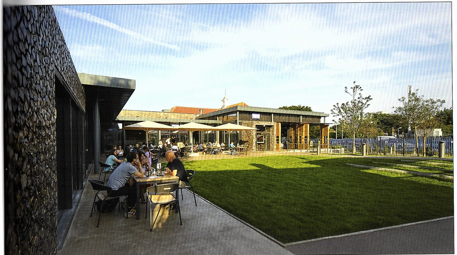
Gallery flint box and north wing to the left, overlooking the paved terrace and lawn. (BFF ©Hufton+Crow.)
