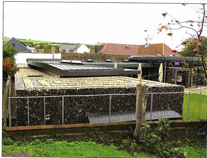
The flint box in the foreground accommodates the gallery while in the background a haze of green marks the downland planted roof over the screens. (David Trevor-Jones.)
