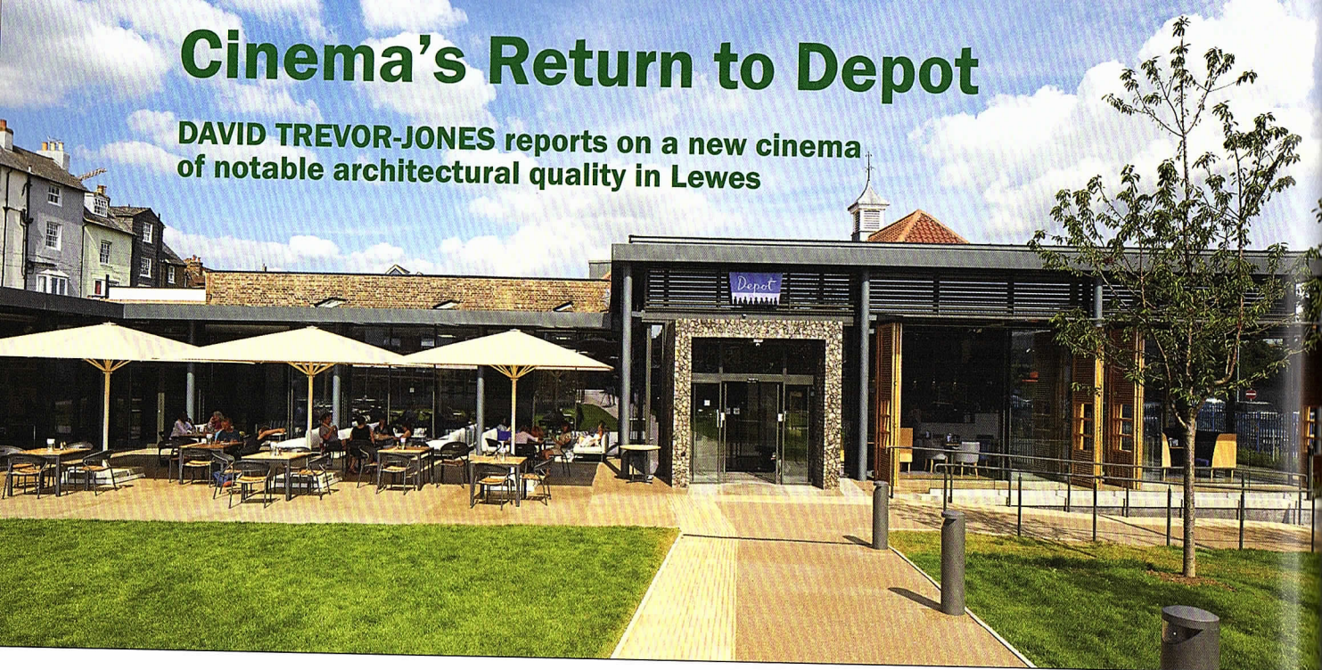
The west wing with entrance aedicule in the centre, café bar to the right and terrace with lounge behind to the left. (Burrell Foley Fischer ©Hufton+Crow.)
