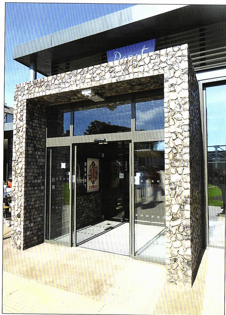
Below: The Flintman's knapped flint entrance aedicule. (David Trevor-Jones.) Right: The flint aedicule punches through the glass. (Carlotta Luke.) Bottom: The box office is a large white desk. Behind it the original brewery depot wall has been retained and train departure times are displayed along with screening information. (David Trevor-Jones.)
